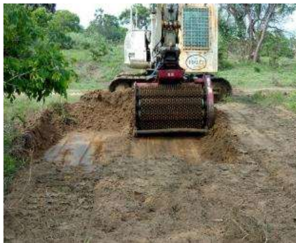
b) Follow up mechanical excavation and filtering
