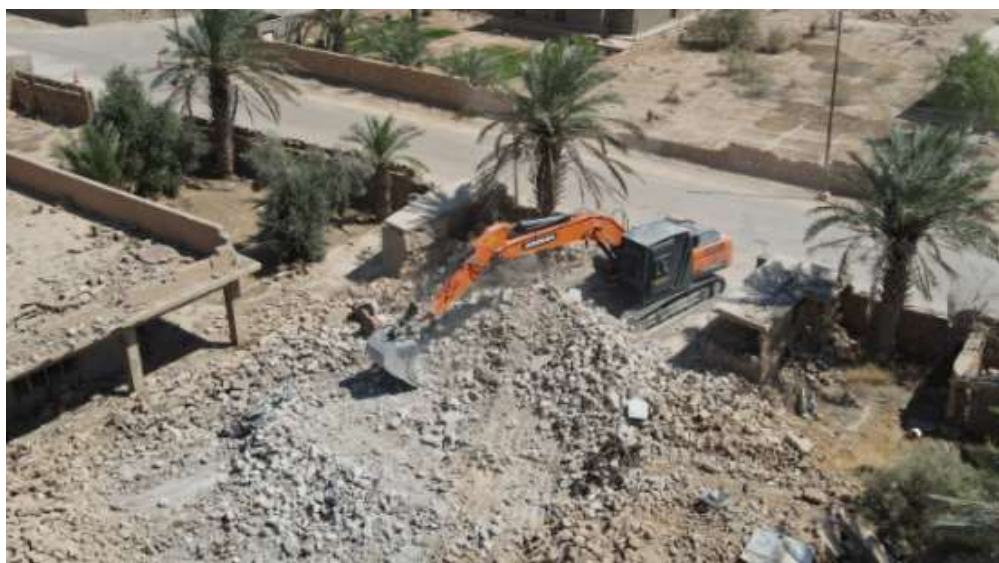
Figure 20 – Tracked excavator with general purpose bucket being used to move rubble to facilitate manual demining – Norwegian Peoples Aid
