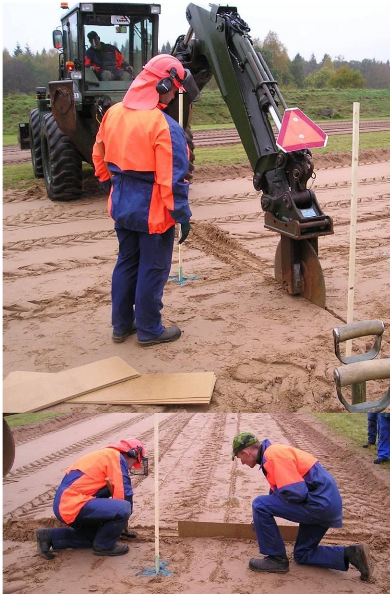
Figure A.3 – Proper fibreboard installation
