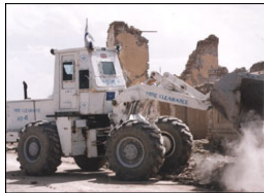
Rubble clearance with armoured front-end loader, Kabul, Afghanistan
